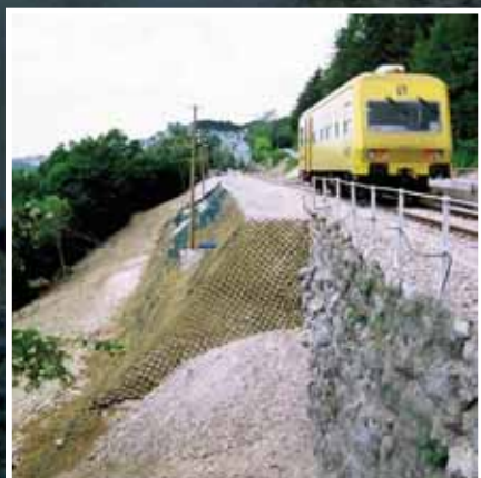
Rehabilitation of retaining wall
