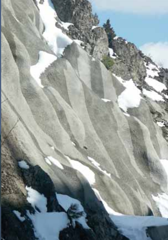
Rehabilitation of the rock with concrete
