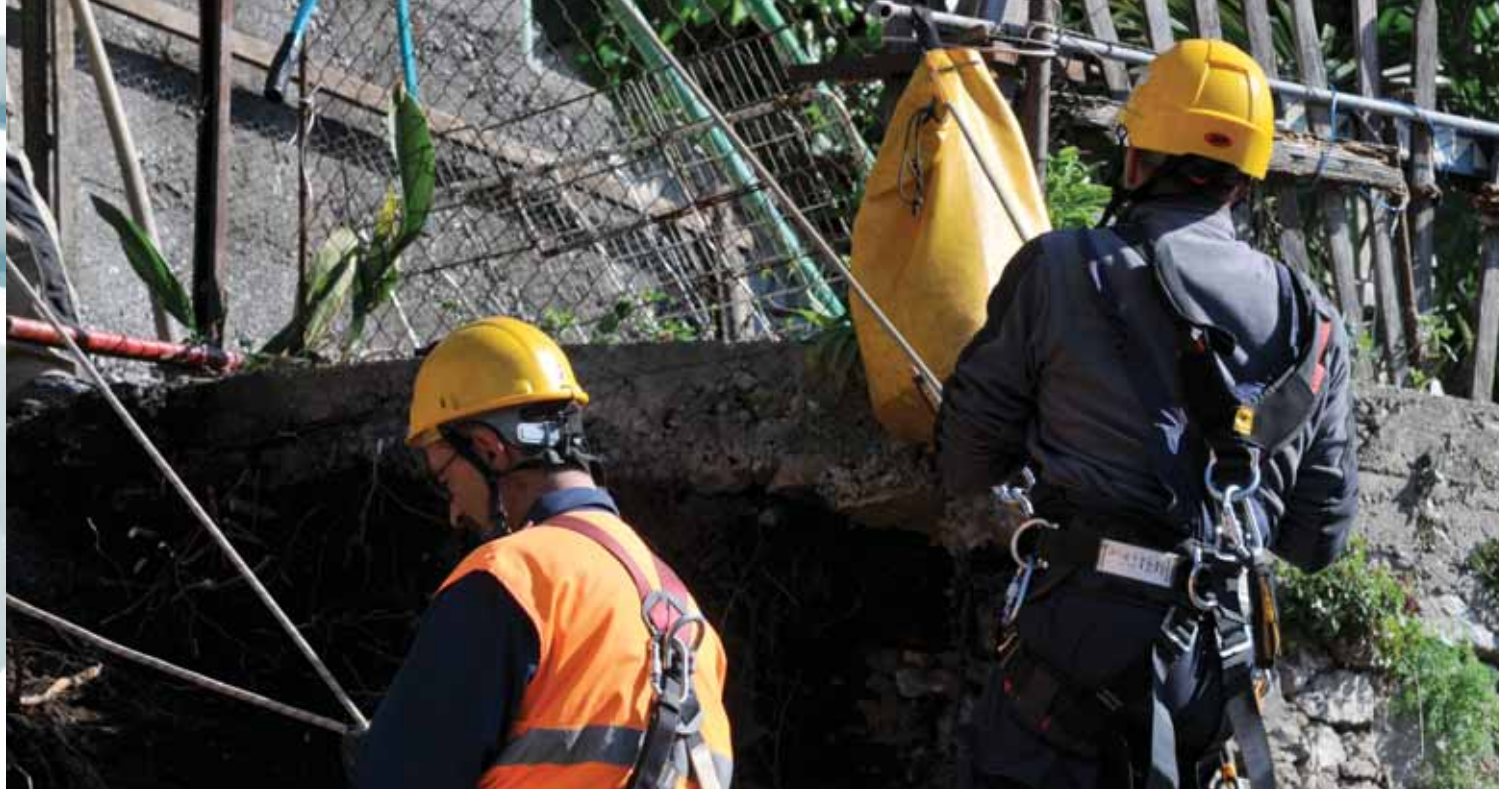
Slope stabilisation at Kalvarija Tunnel
